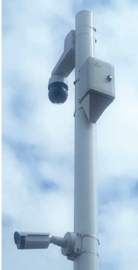
Danger recognition: A Slat Synaps 24V 3E IP with a built-in 60W high PoE injector and a fiber-optic media converter supplying and buffering moveable Axis dome infra-red cameras
