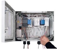
The Synaps-PoE is an outdoor network interface box dedicated to video applications and PoE powered transmissions, ensuring continuity of service for the equipment it protects
